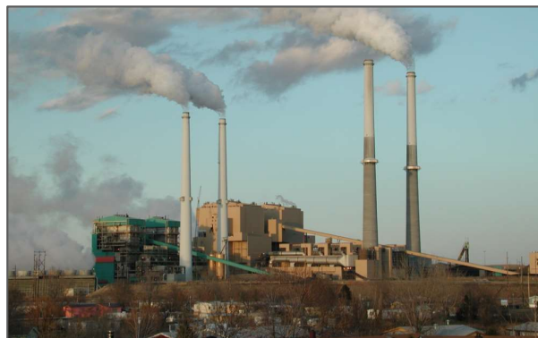
Owned Energy Supply
