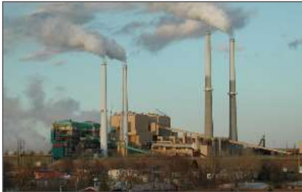
Owned Energy Supply
