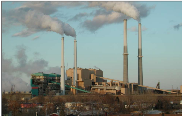
Owned Energy Supply
