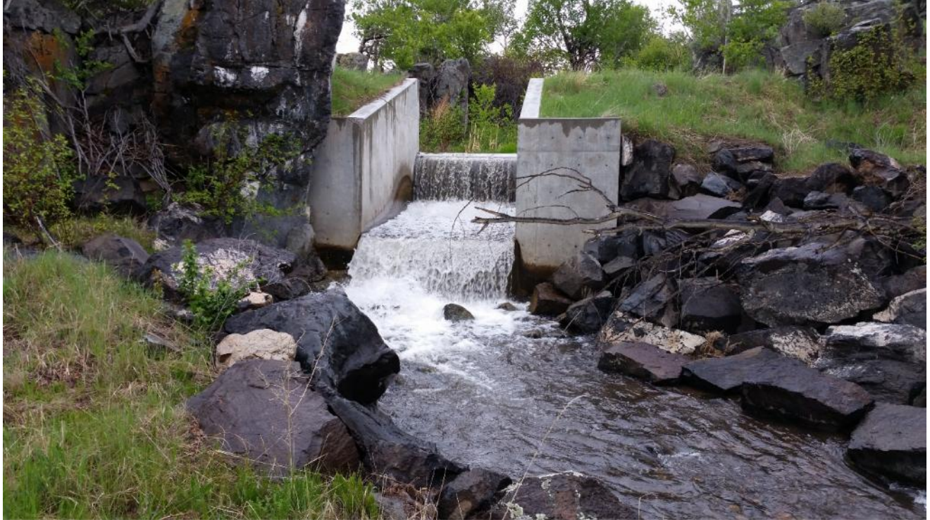
Photo 1. Barrier on Cherry Creek near Melrose, MT which is similar in design to the French Creek barrier.
