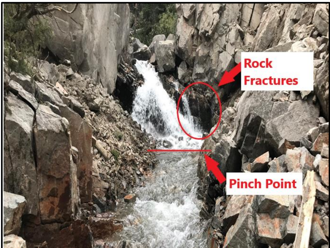
Figure 20. Tepee Creek barrier and potential points of failure.
