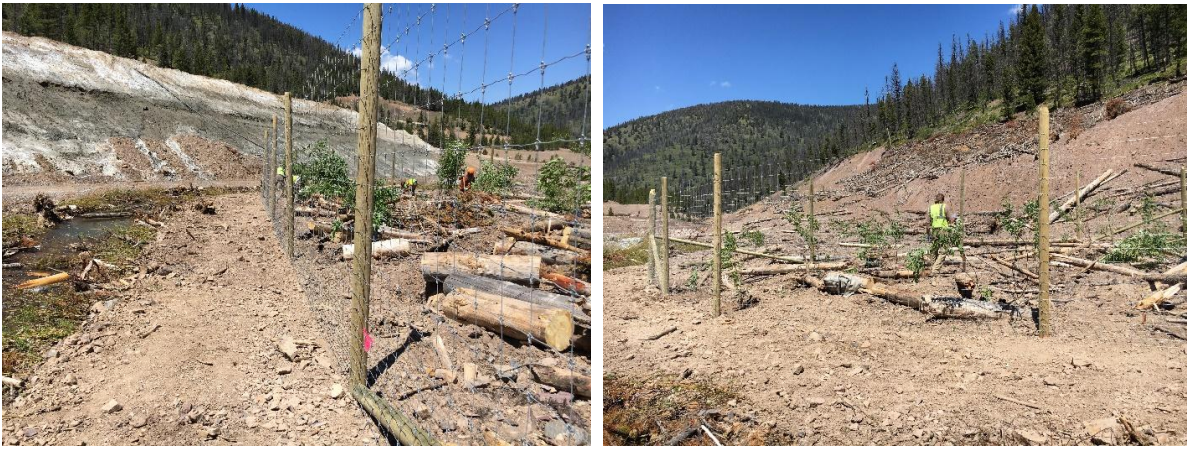
Figure 1. Example of a wildlife exclosure fence installed at restoration site near Lincoln, Montana.
