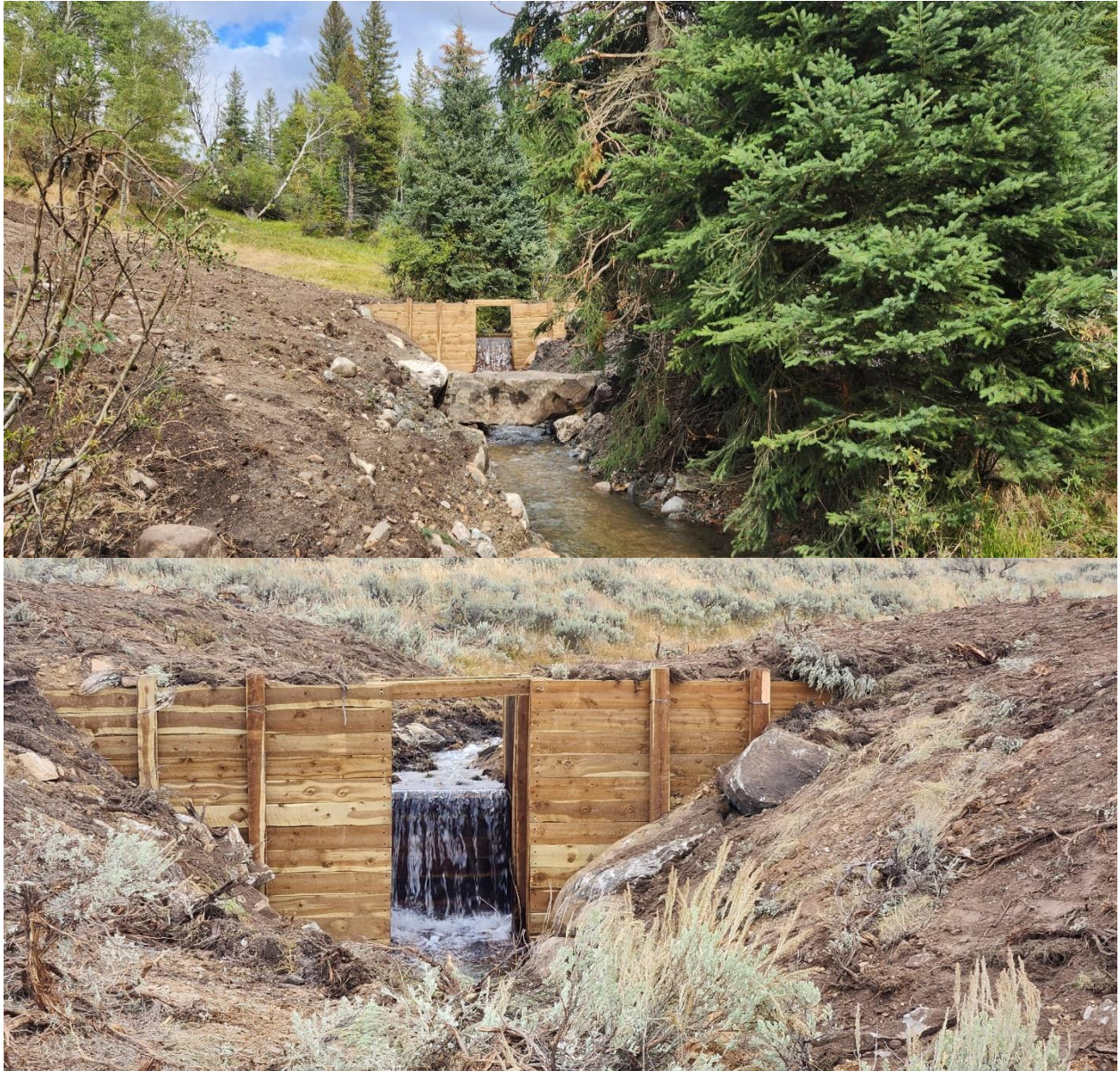
Figure 17. Wooden migration barriers installed on Pine Butte (top photo) and Deadman (bottom photo) creeks in 2022.
