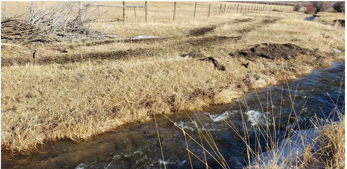
Figure 22. - Berm material removed to reconnect flood plain.
