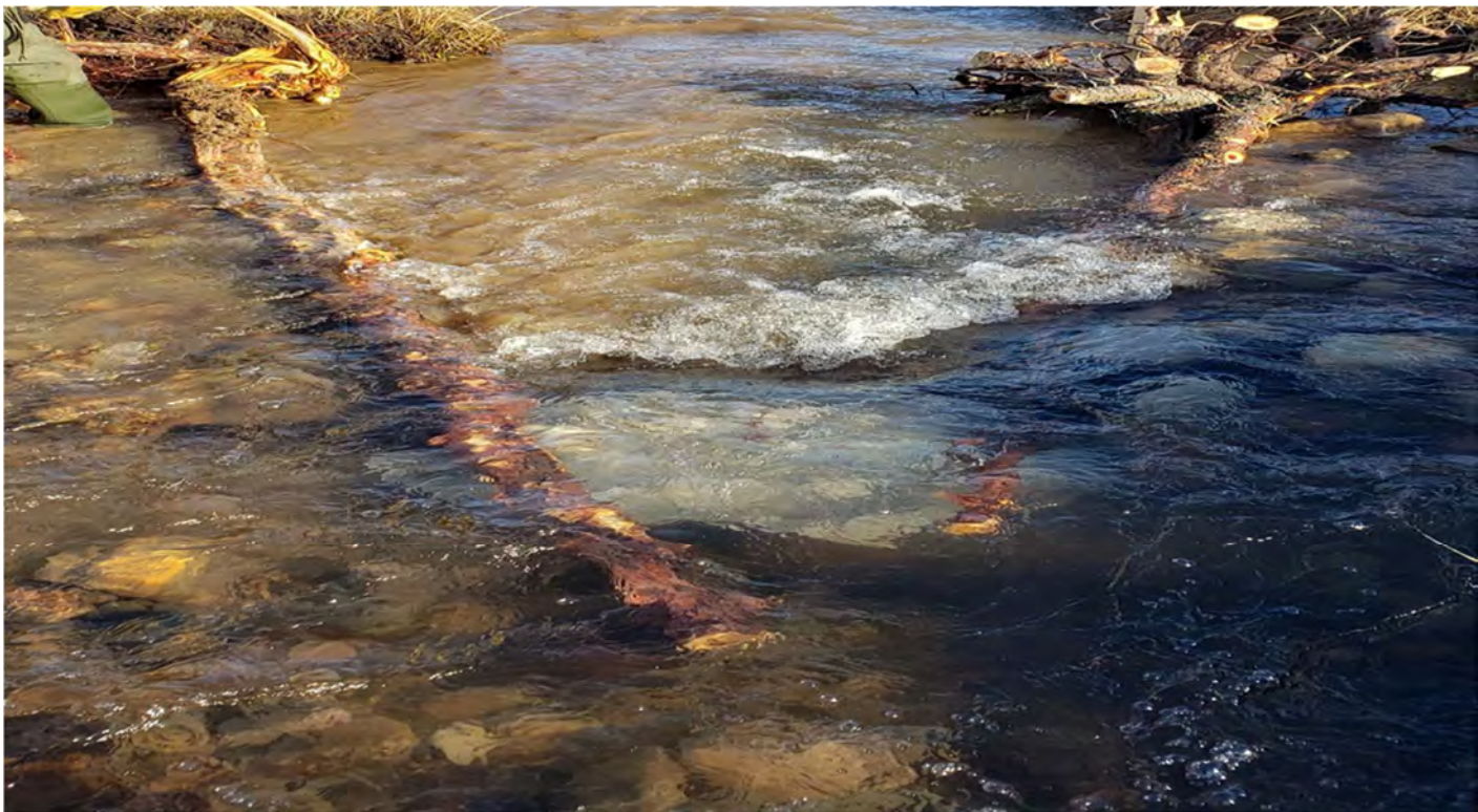
Figure 23.- Placement of instream structure for pool development.
