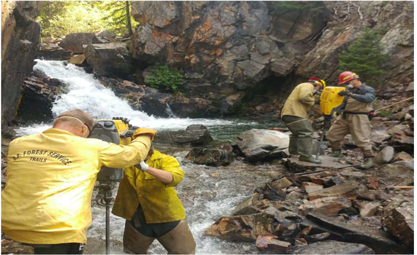
Figure 17.- Custer-Gallatin National Forest explosives crew preparing to blast bedrock to enhance fall on Tepee creek for a migration barrier. Photo courtesy of Allison Stringer Custer-Gallatin National Forest Service.
