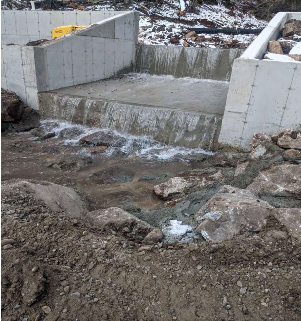
Figure 18. Completed Wall Creek barrier in November 2021.
