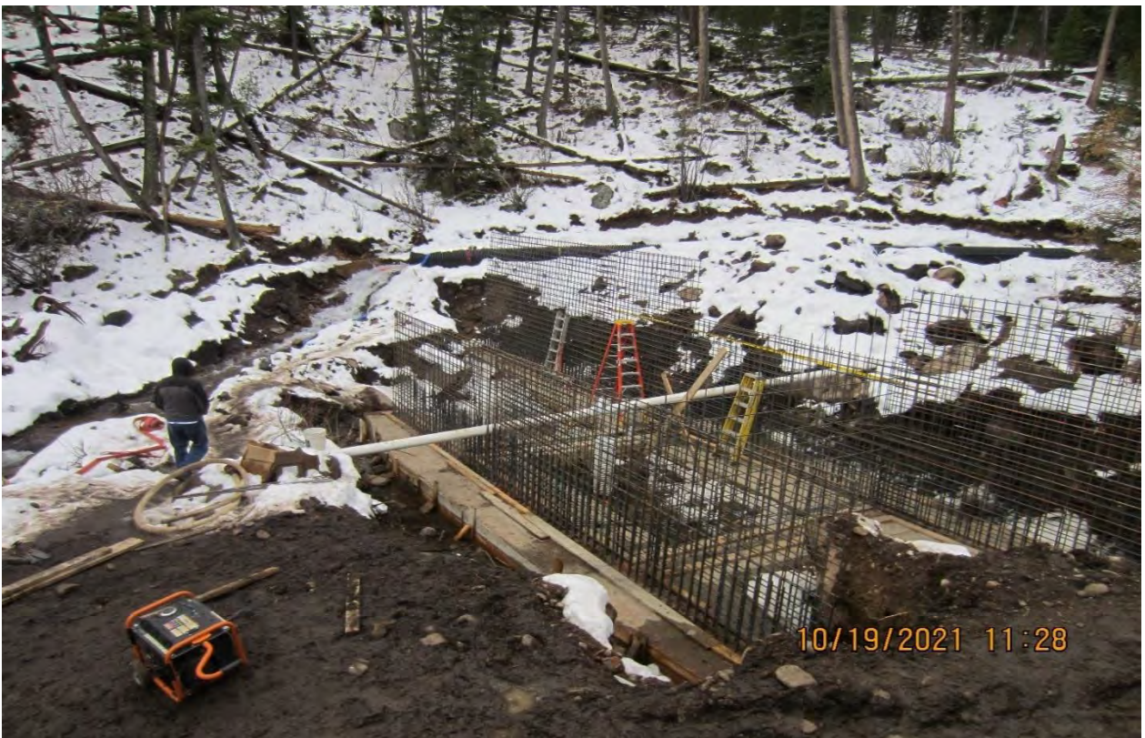
Figure 17. Wall Creek concrete barrier forms.
