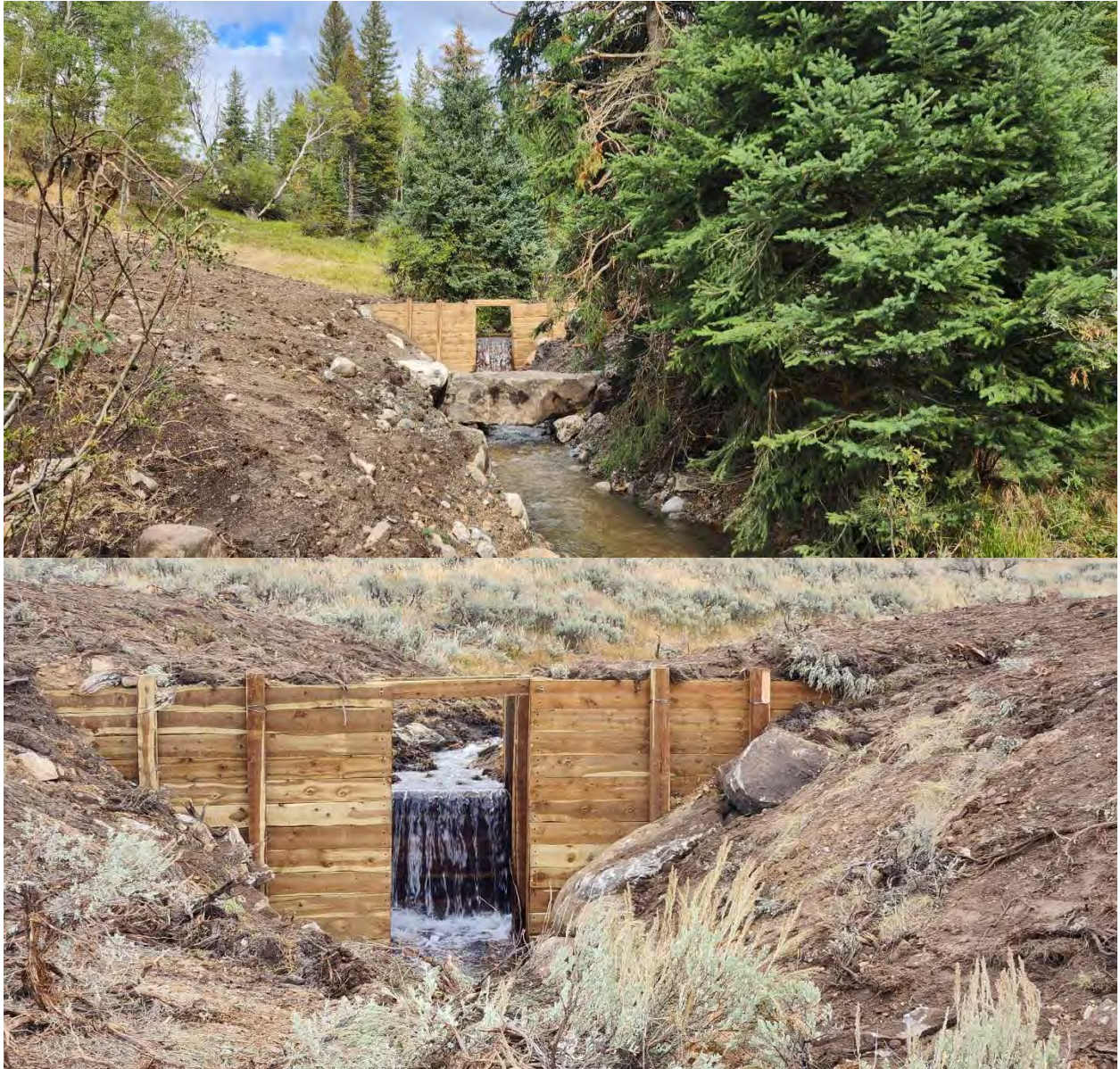
Figure 17. Wooden migration barriers installed on Pine Butte (top photo) and Deadman (bottom photo) creeks in 2022.
