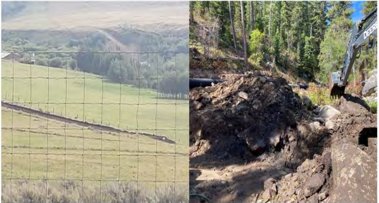
Figure 16. Road improvements and barrier site excavation on Wall Creek.
