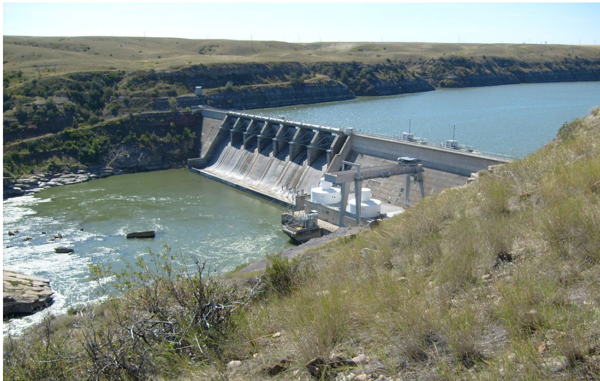
Figure 2-4. Photograph of Cochrane Dam
