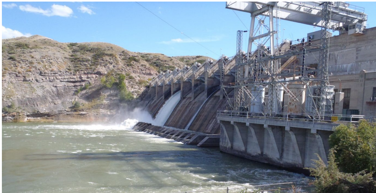
Figure 2-6. Photograph of Morony Dam
