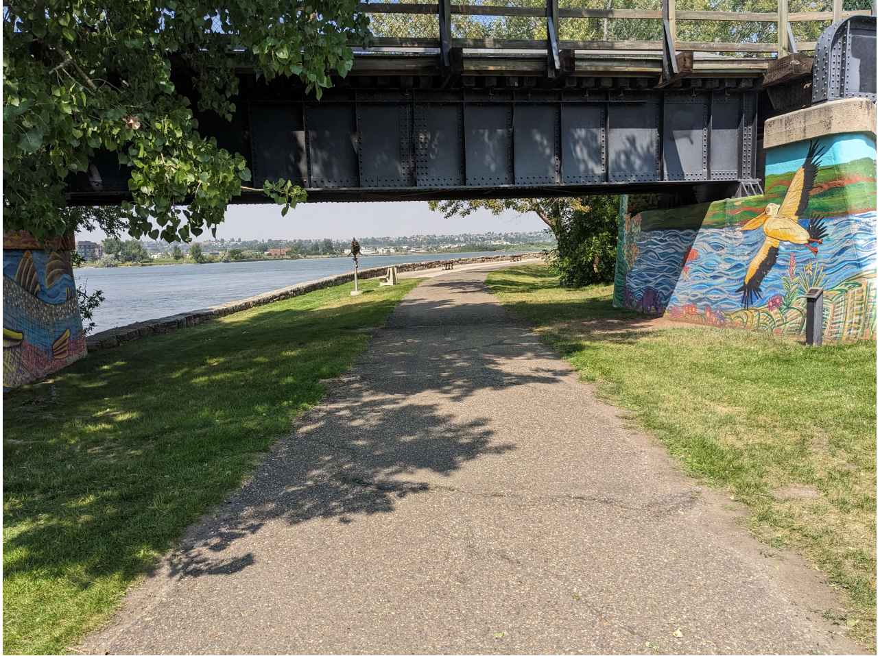
Current asphalt trail surface condition photos
