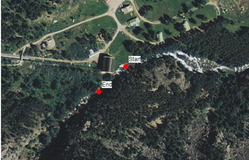
Figure 9: West Rosebud Creek Lower Bypass Section location. Start coordinates: 45.24345 N, -109.7319 W. End coordinates: 45.24305 N, -109.7325 W.
