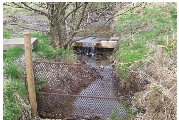
Settling Basin and Trash Rack
