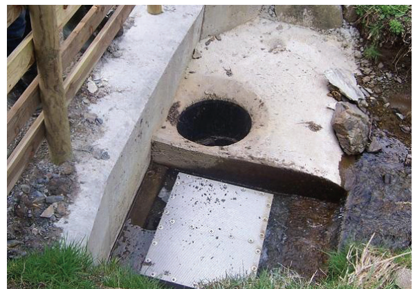
Forebay and Submerged Penstock Entry
