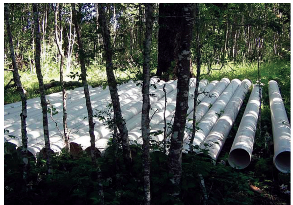
PVC Pipe Ready for Joining and Burying
