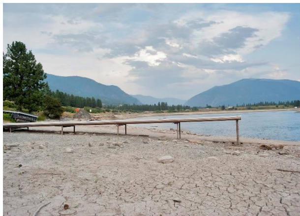
Draw down of Thompson Reservoir left shoreline and access areas void of water for much of July and early August to facilitate work on the Main and Dry Channel Dams. Photo credit: Linda Elliott.
