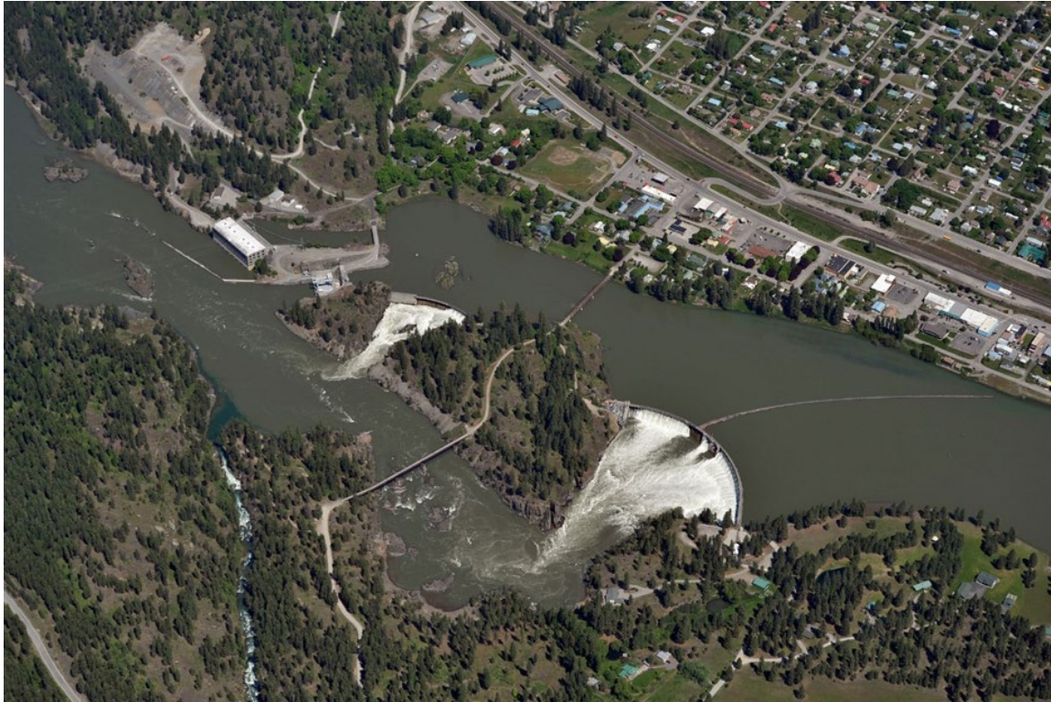
Photograph 7-2: Aerial of Thompson Falls Hydroelectric Project and Prospect Creek, June 2017.
