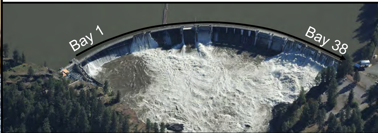
6 Panels per Bay
