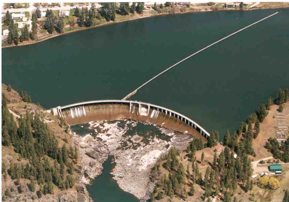
Figure 3 – Aerial photo of Main Dam Spillway.
