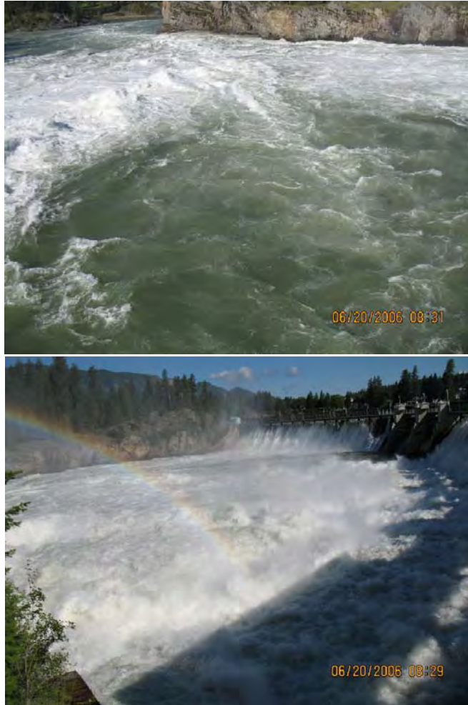
Figure 3-8. Thompson Falls Main Dam Tailrace.
