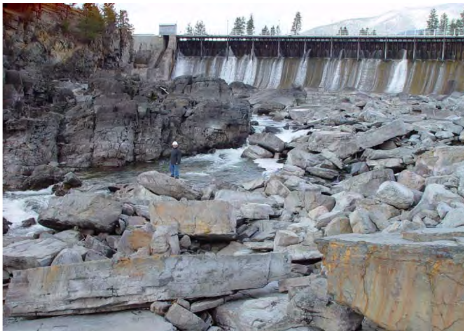
Figure 4 – Steep center thalweg and “falls” roughness.
