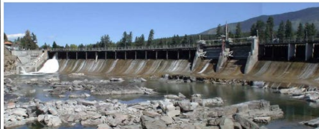
Right Side of Dam
