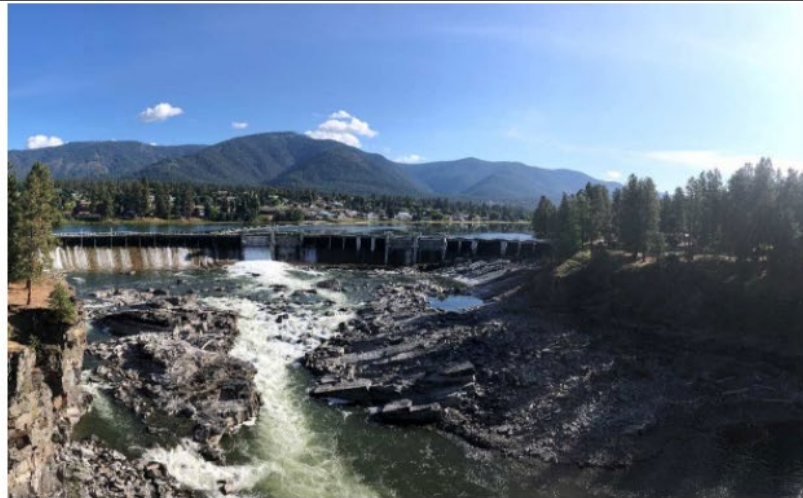
Looking Upstream Towards Dam
