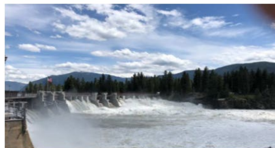
Left Side of Dam
