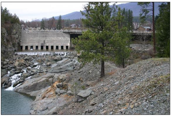
MT\_SandersCounty\_ThompsonFallsHydroelectricDamHistoricDistrict\_00010 Dry Channel Dam, downstream side, with non-overflow waste gate structure at left, camera facing north.
