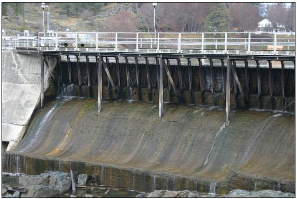
MT\_SandersCounty\_ThompsonFallsHydroelectricDamHistoricDistrict\_0011 Dry Channel Dam overflow section, showing flashboard (bottom) and drop panel (top) gates, camera facing northwest.
