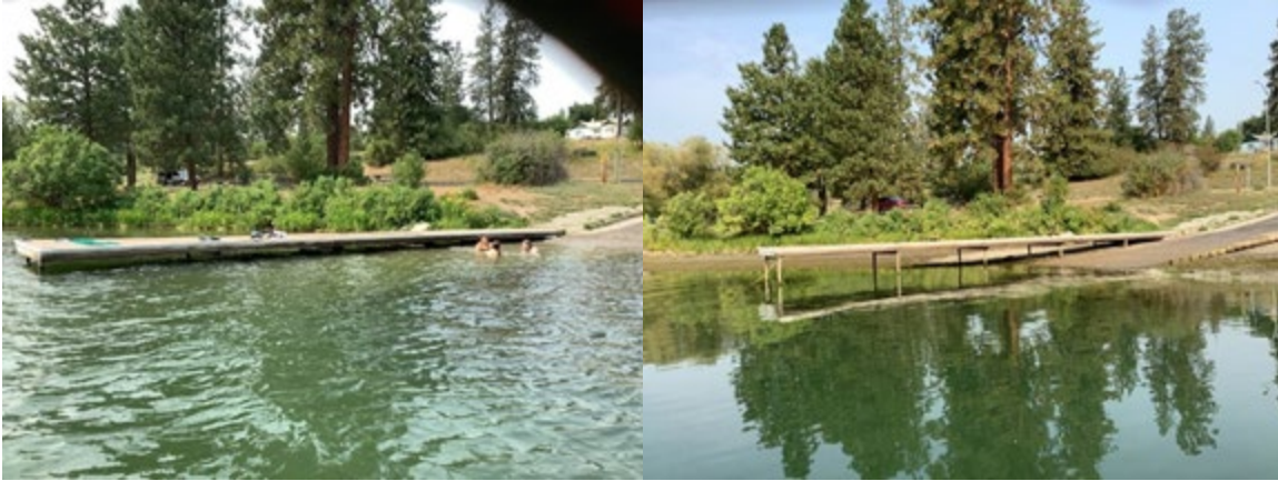
Wild Goose Landing stationary boat launching dock, north shore main reservoir, at full pool and -2.5 feet elevation.
