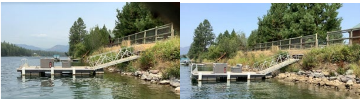
North shoreline floating dock at full pool and with steep gangway angle at -1.5 feet elevation.
