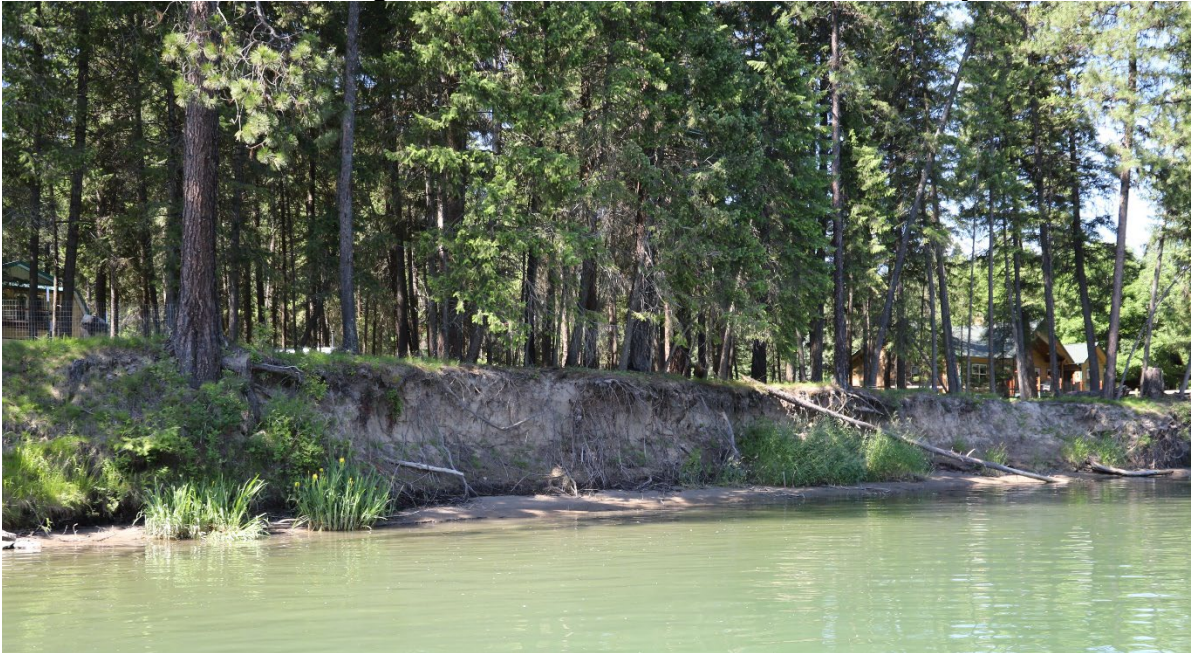
Photo 3-6. Photos of Eroding Bank Before Shoreline Stabilization Pilot Project
