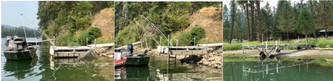
North shoreline stationary dock with boat whips at full pool and -2.0 feet elevation, and south shoreline stationary dock mostly dewatered at -2.5 feet elevation.
