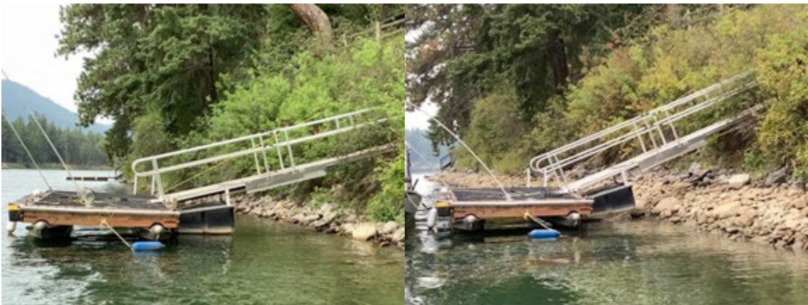
North shore floating dock at full pool and with very steep gangway at -2.5 feet elevation.
