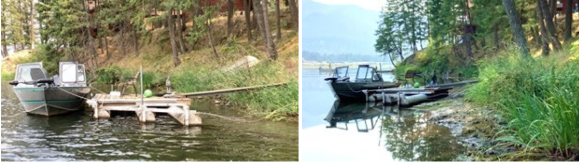
South shoreline main reservoir floating dock at full pool and mostly dewatered at -1.5 feet elevation.
