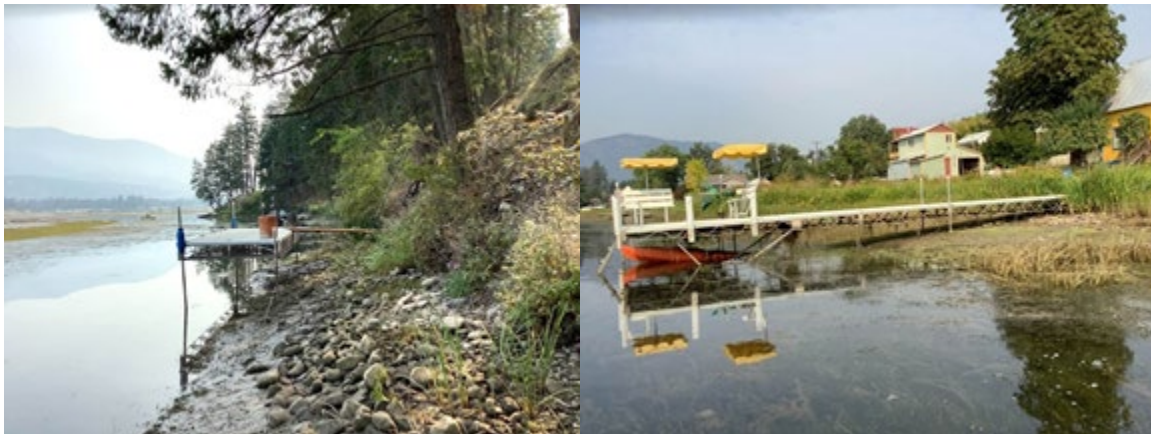
South shoreline main reservoir stationary dock North shoreline main reservoir stationary dock mostly dewatered at -2.5 feet elevation with aquatic vegetation at -2.5 feet elevation.
