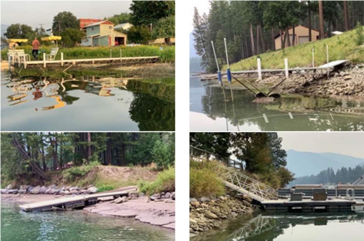
Photos 3-20: Impacts to Dock Access at Varying Water Elevations.
