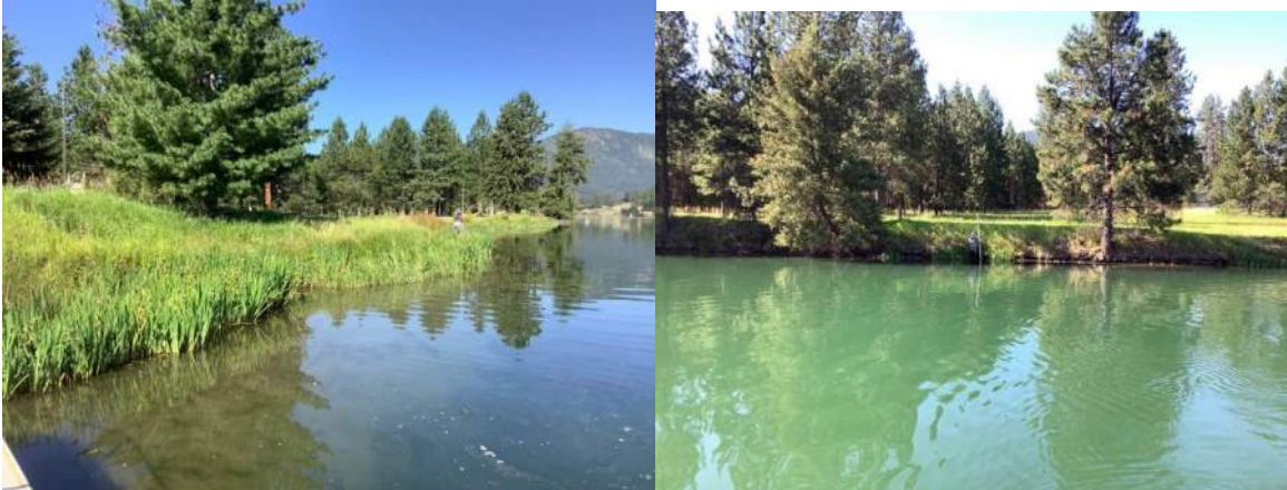
Bank profile looking downstream from mid-point, and upper 100 feet of the 300-foot reach.
