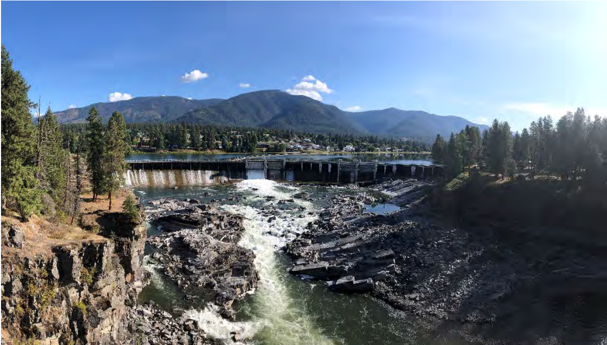
Photograph 2-2: Thompson Falls Project Main Channel Dam, with the new radial gates. (Photo: Kim Bergstrom, Pinnacle Research.)
