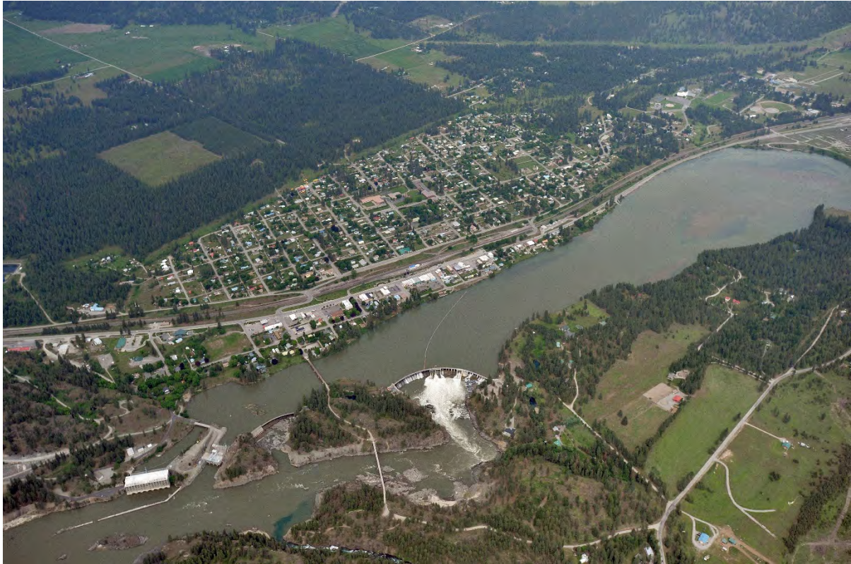
Photograph 2-1: Aerial photo of the Thompson Falls Project looking upstream.
