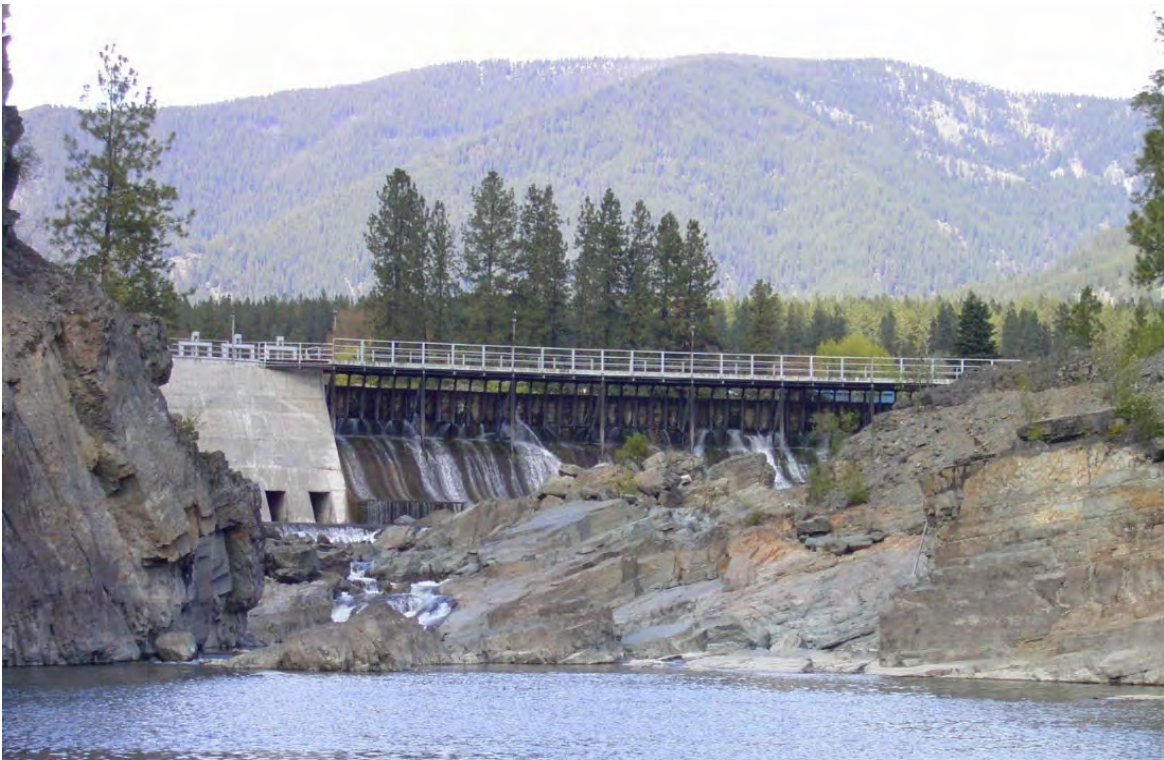
Photograph 2-3: Dry Channel Dam.
