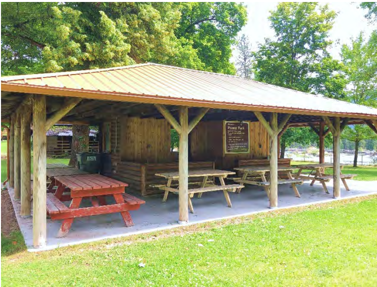
Photographs 9-6: Information kiosk (top); trail access at edge of park (middle left); restroom (middle right); group use portion of pavilion (bottom).
