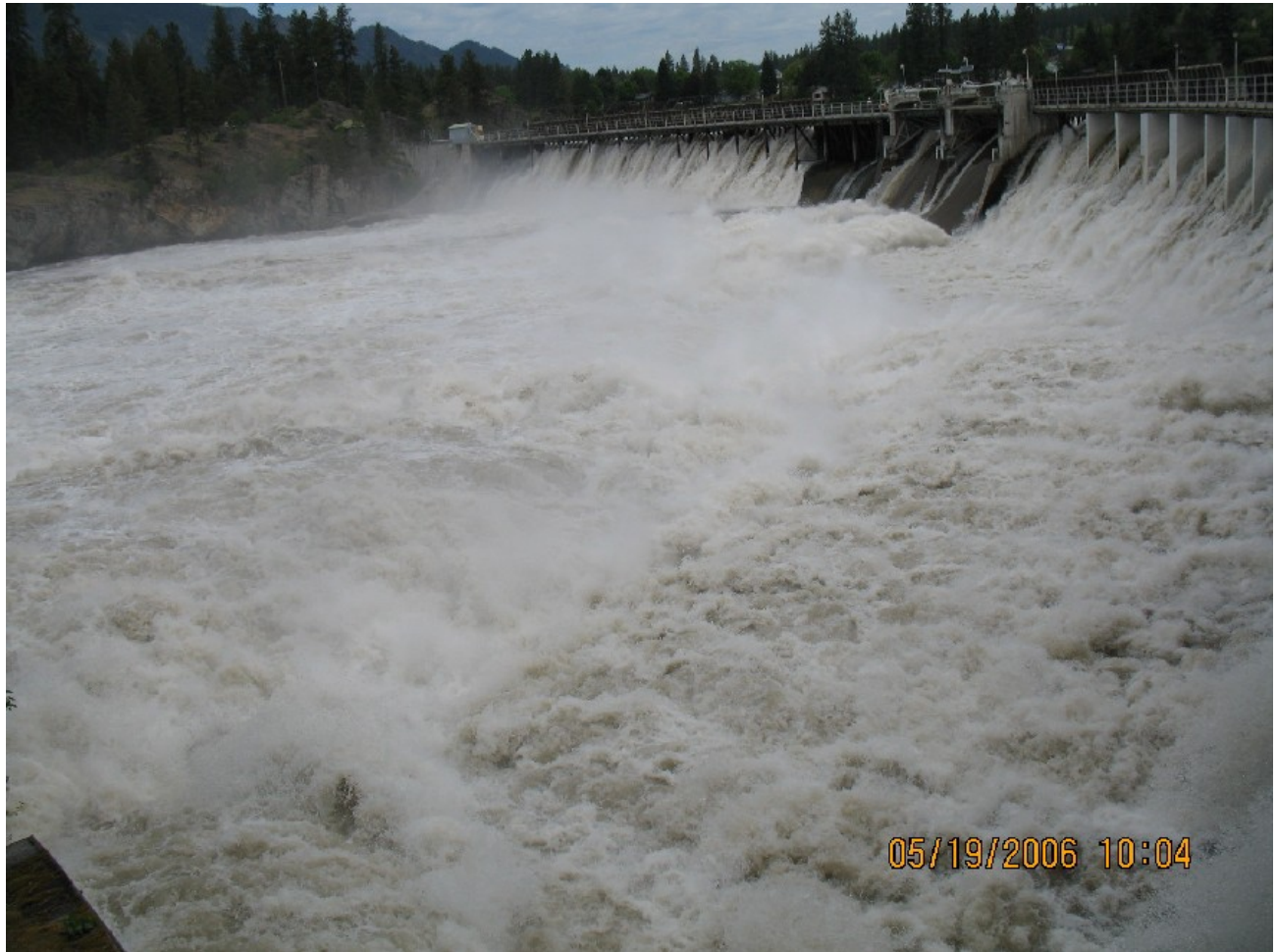
Figure 12-2: Photographs of the Clark Fork River downstream of the Main Channel Dam at high flow (between 68,400 and 76,450 cfs)
