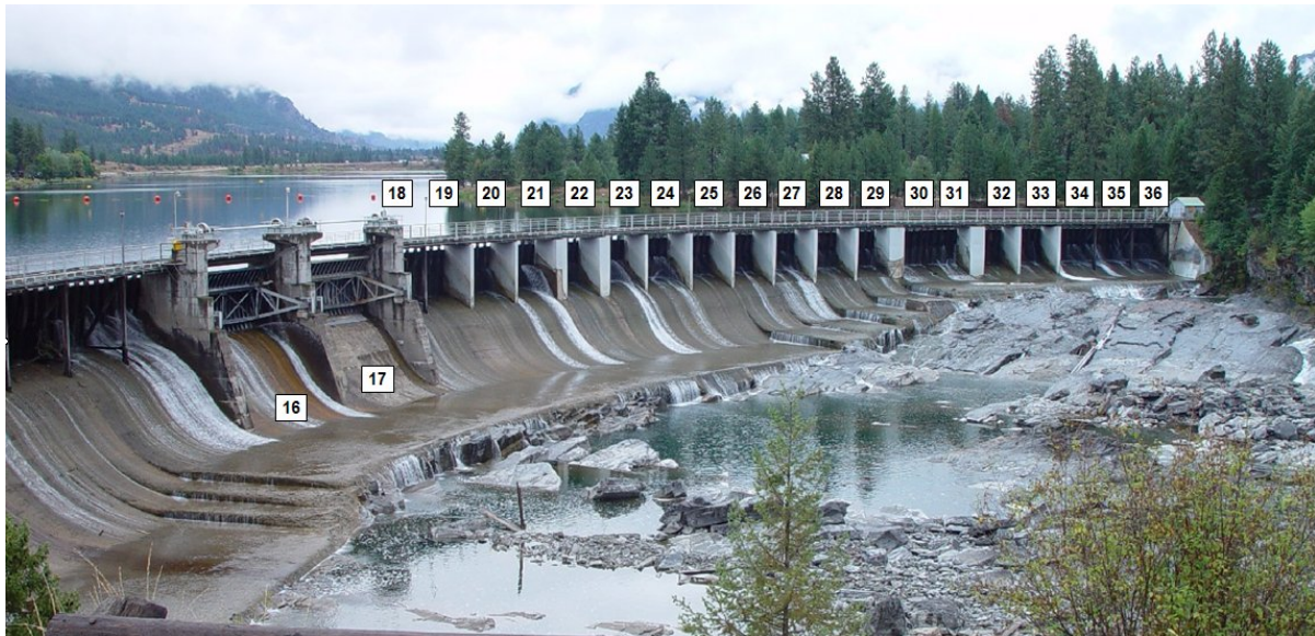
Photo 6-2: The left bank of the Main Dam at the Thompson Falls Project, with the spillway bays numbered.
