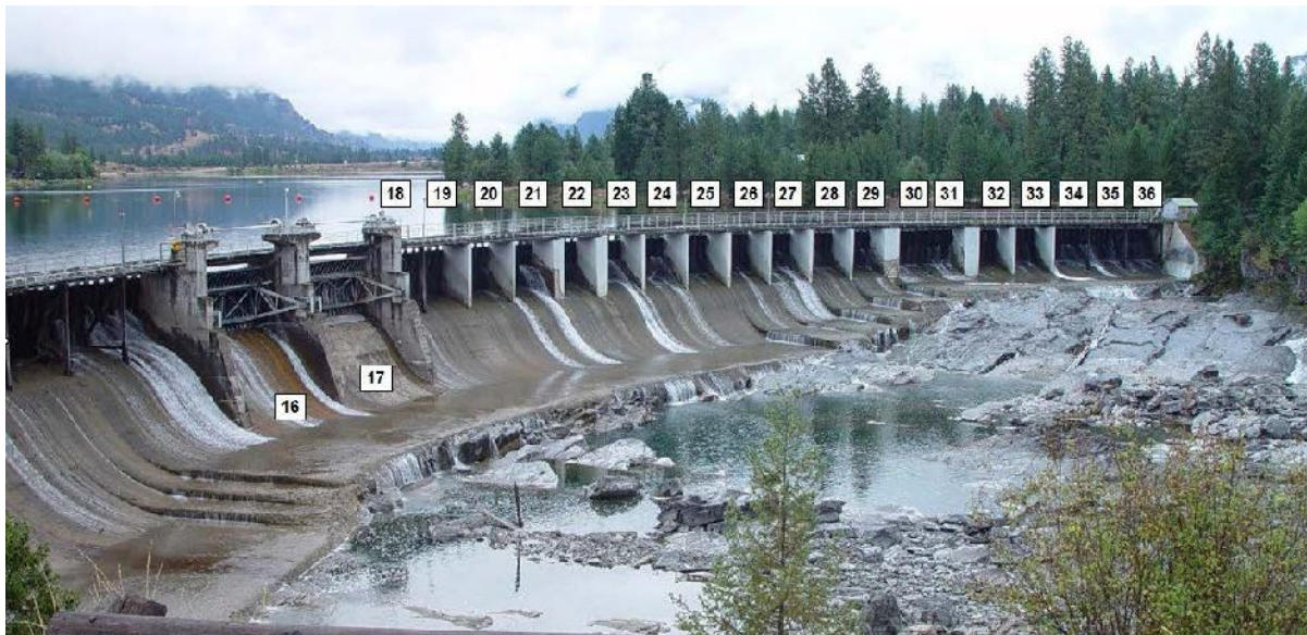
Photo 7-2: The left bank of the Main Dam at the Thompson Falls Project, with the spillway bays numbered.
