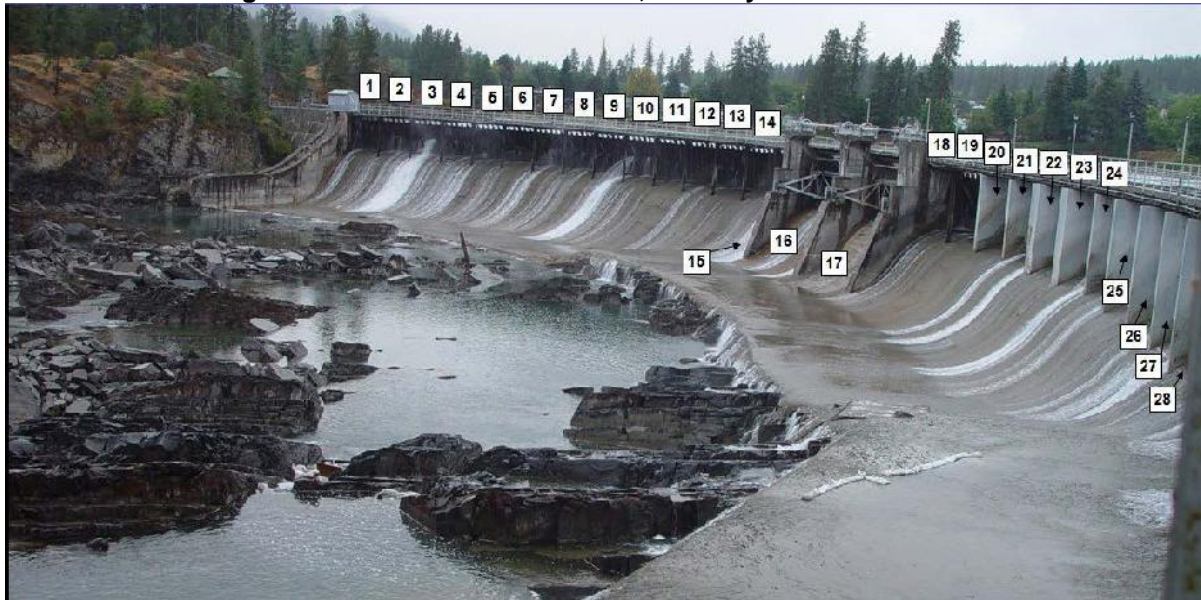
Photo 7-1: The right and center of the Main Dam, with bays numbered.
