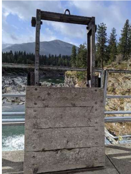
Photograph 1. Panel with boards removed for attraction flow.
