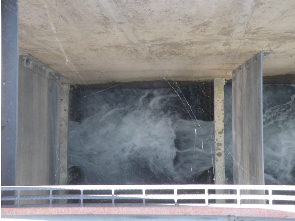
Photo 5: Plunging pool-to-pool weir flow typical of Lower Ladder pools
