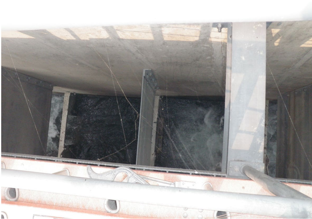
Photo 12: Pool-to-pool overflow weir flow in lower ladder pools.
