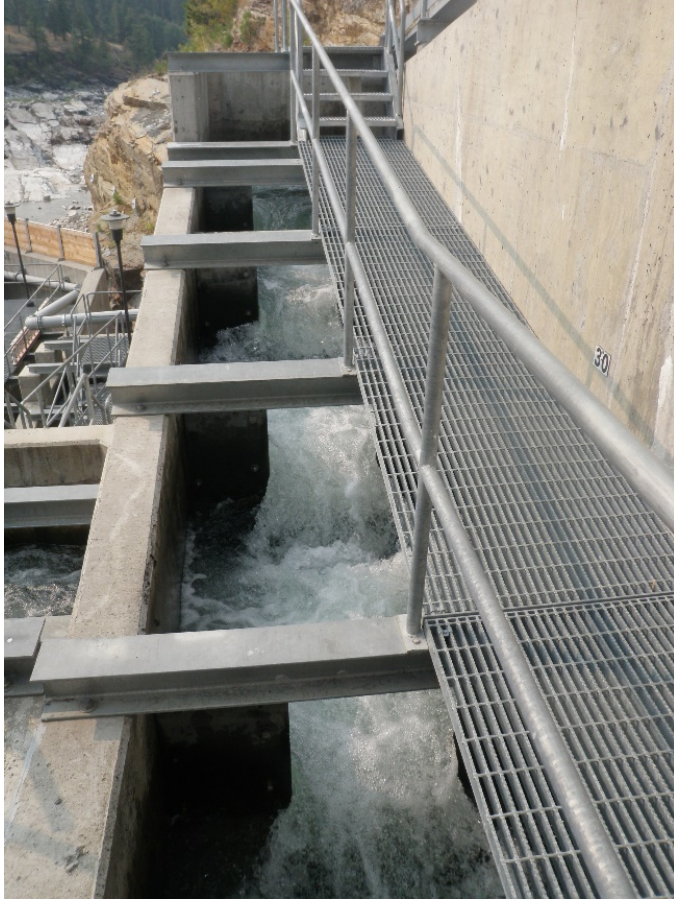
Photo 11: Pools 29 through 34 operating in overflow weir mode. Based on field measurements, weirs 29/30 and 30/31 exhibited pool to pool flow with about 0.3 feet of weir submergence and a differential of approximately 0.6 feet between each pool.
