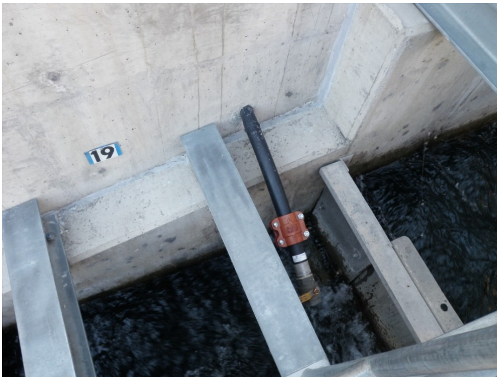
Photo 3: Transition from turning pools to lower ladder straight pool section. This weir had the largest pool-to-pool drop of the ladder when operating in orifice mode.
