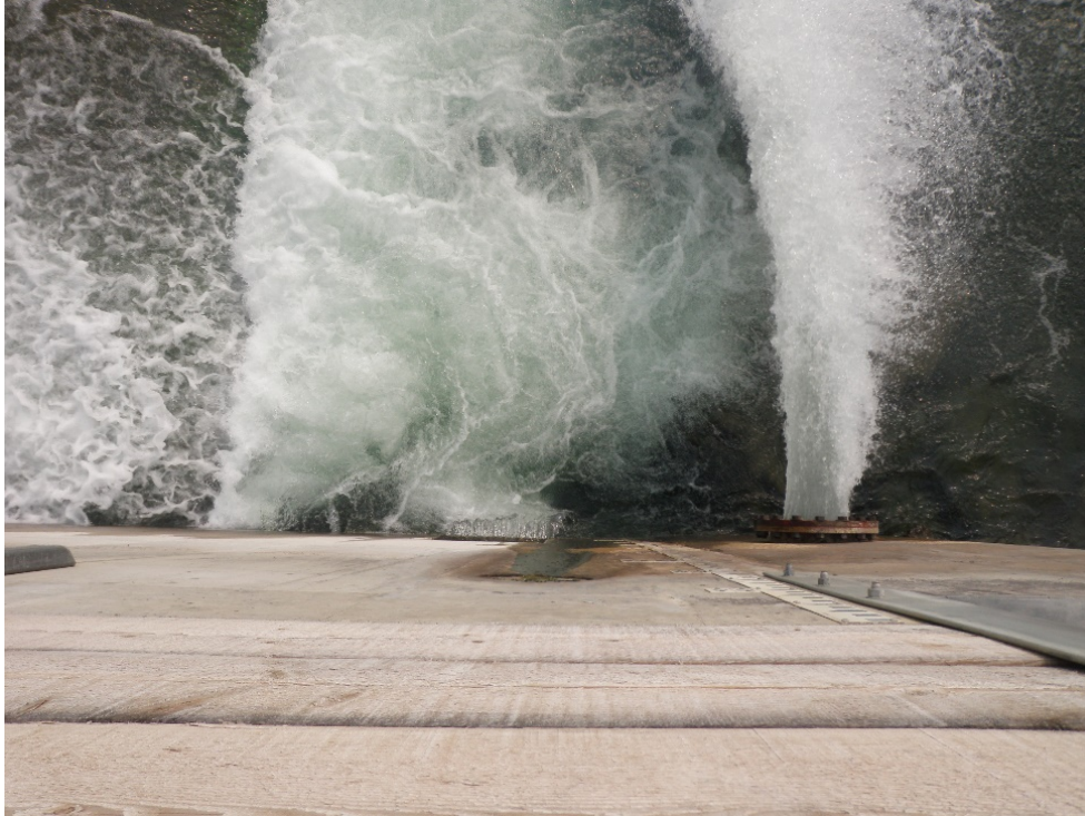
Photo 13: Conditions at Entrance Pool with high velocity attraction jet at right. Note both gates fully open and several inches of flow was passing over the upper gate.
