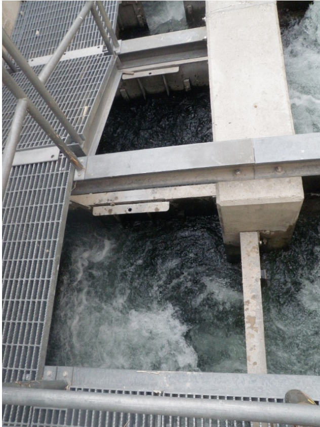
Photo 7: Pool 9 (lower left) and Pool 8 (mid-left) operating in orifice mode for use with PIT tag readers. Water level differential between Pools 9 and 10 was only 0.21 feet due, in part, to the presence of the PIT tag antenna.
