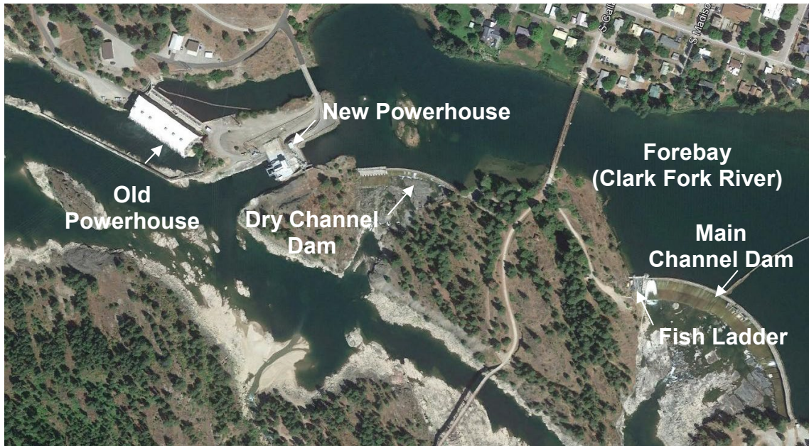
Figure 1: Thompson Falls Hydroelectric Project (Google Earth 2017)
