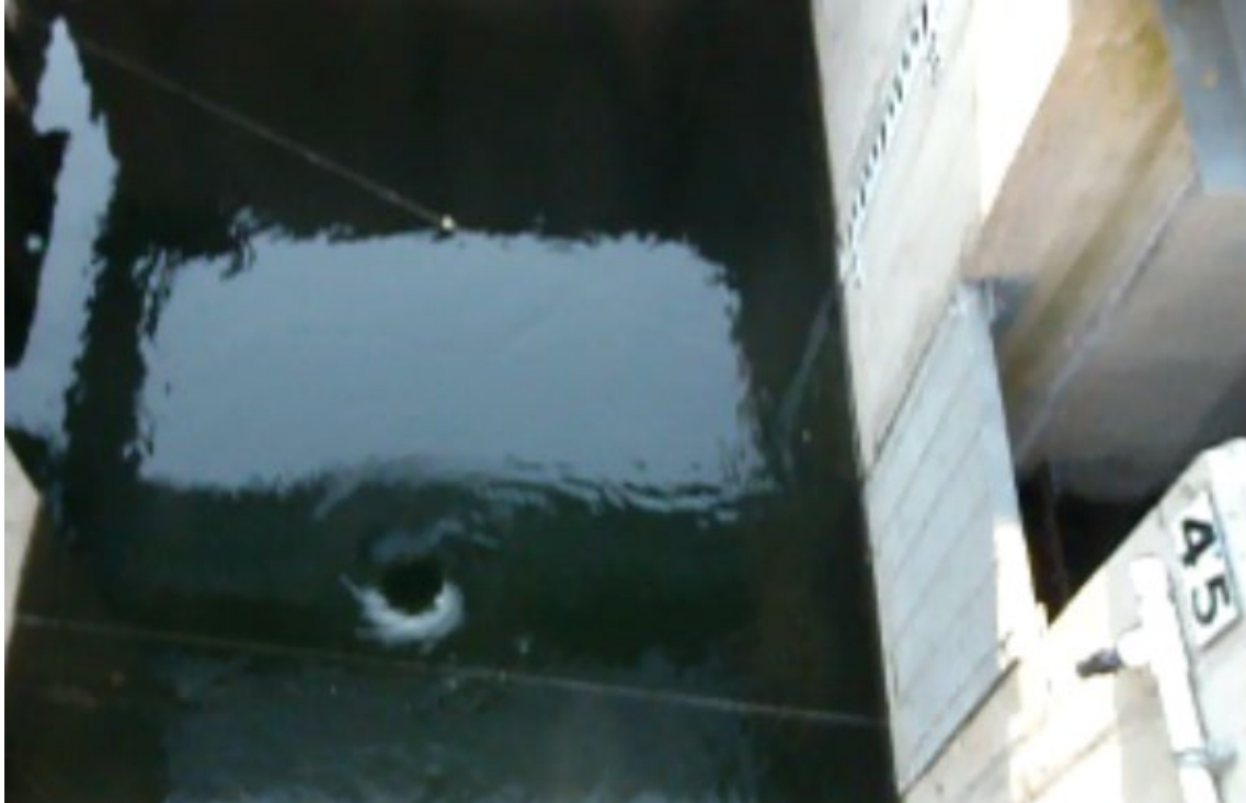
Photo 1: Vortex observed in pool 45 near bleed-off diffuser.
