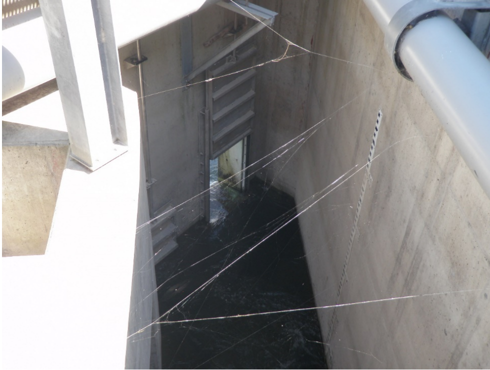
Photo 6: Conditions at Entrance Pool with both gates fully opened
