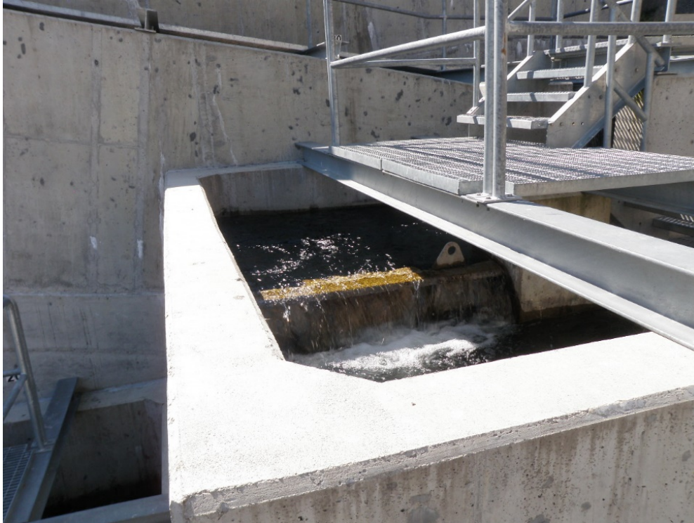
Photo 4: Overflow at Pool 26/27 Weir Operating in Orifice Mode
