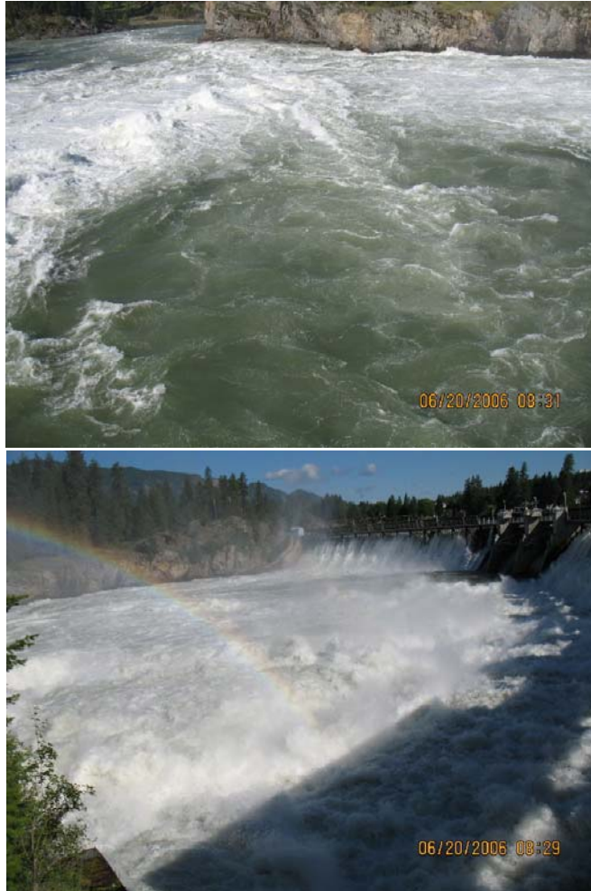
Figure 3-8. Thompson Falls Main Dam Tailrace.
