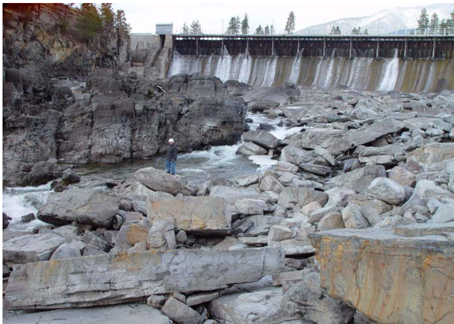
Figure 4 – Steep center thalweg and “falls” roughness.
