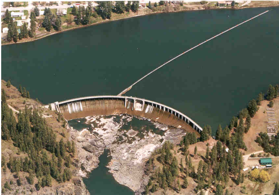
Figure 3 – Aerial photo of Main Dam Spillway.
