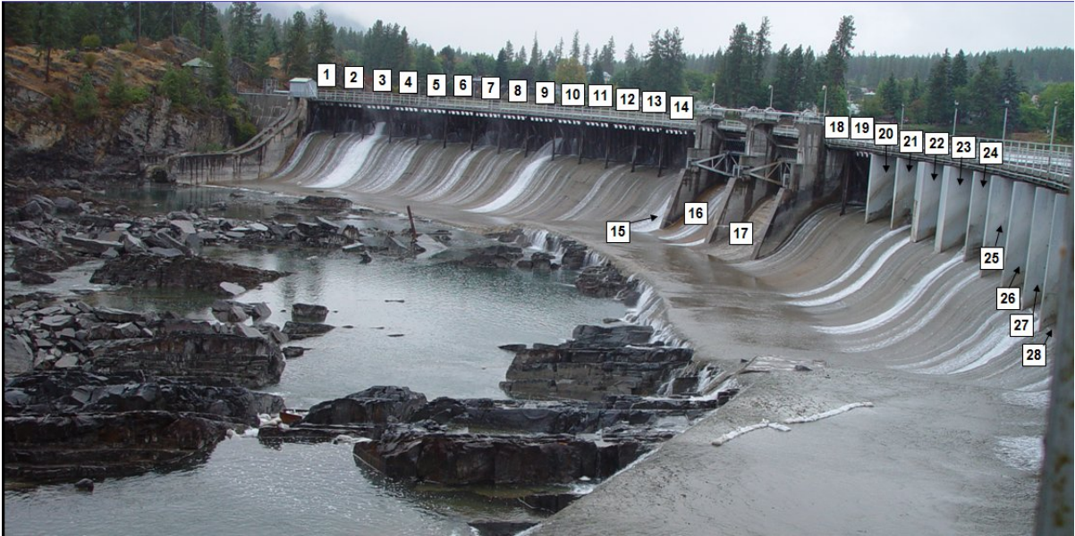
Photo 1. The right and center of the Main Dam, with bays numbered.
