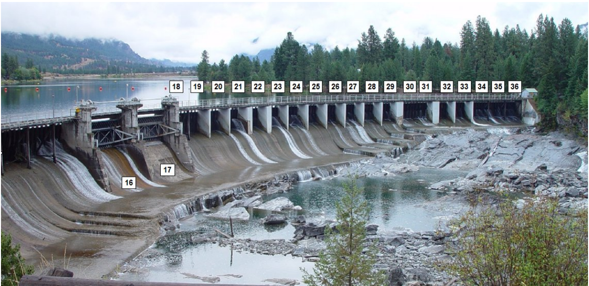
Photo 2. The left bank of the Main Dam at the Thompson Falls Project, with the spillway bays numbered.
