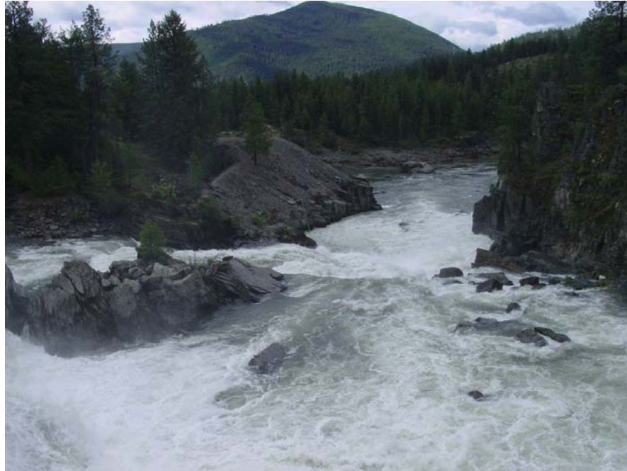
Figure 3-17. Three photos taken during 2010, with water passing through the Dry Channel. Photos were taken July 2, 2010 when all 12 bays were pulled out on the Dry Channel Dam and total flow was about 45,000 cfs. The second photo shows the current from the Dry Channel Dam shooting across the main river channel to hit the far bank near where Prospect Creek empties into the Clark Fork.
